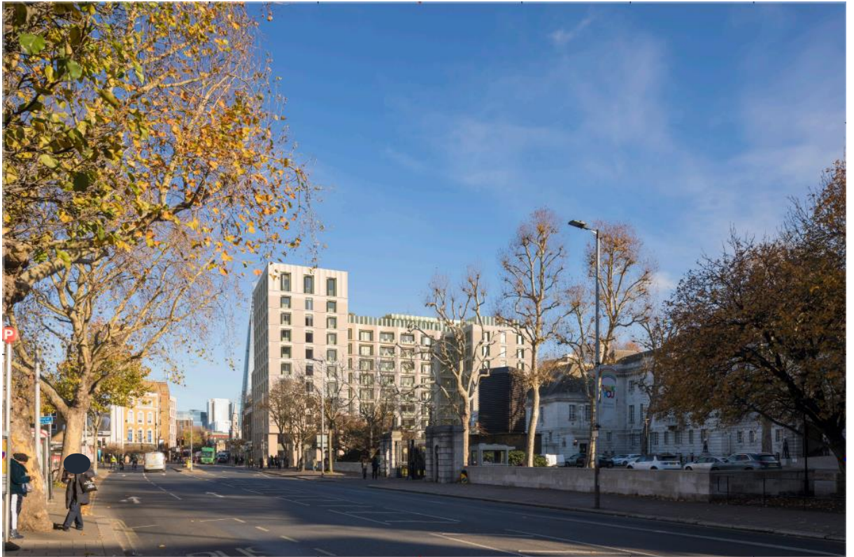
View to the north with the Inner London Court (Grade II listed) on the right
